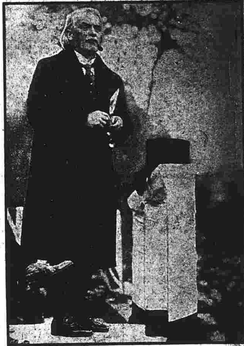
During his stay in the Dominion, Lloyd George turned the sod for a new Baptist church at Westmount, Canada, and then delivered a speech to an eager crowd.
